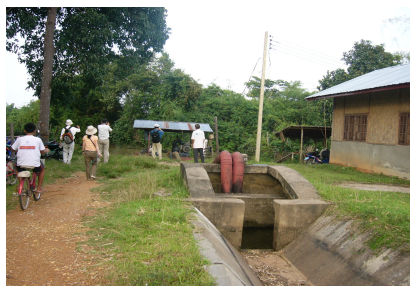
Napho Tai地区：Decentralized Irrigation Development and Management Sector Project (DIDMSP) の視察。幹線水路と奥が河川。
