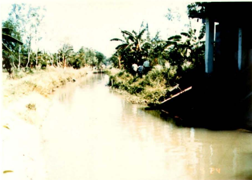
Sinocalan River Irrigation System Main Canal
