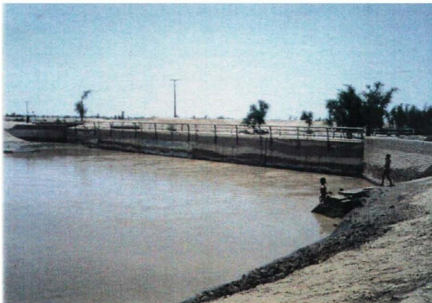
Structure to divert hill torrent into the Indus River
