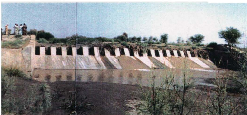
View of Spill weir to control hill torrent
