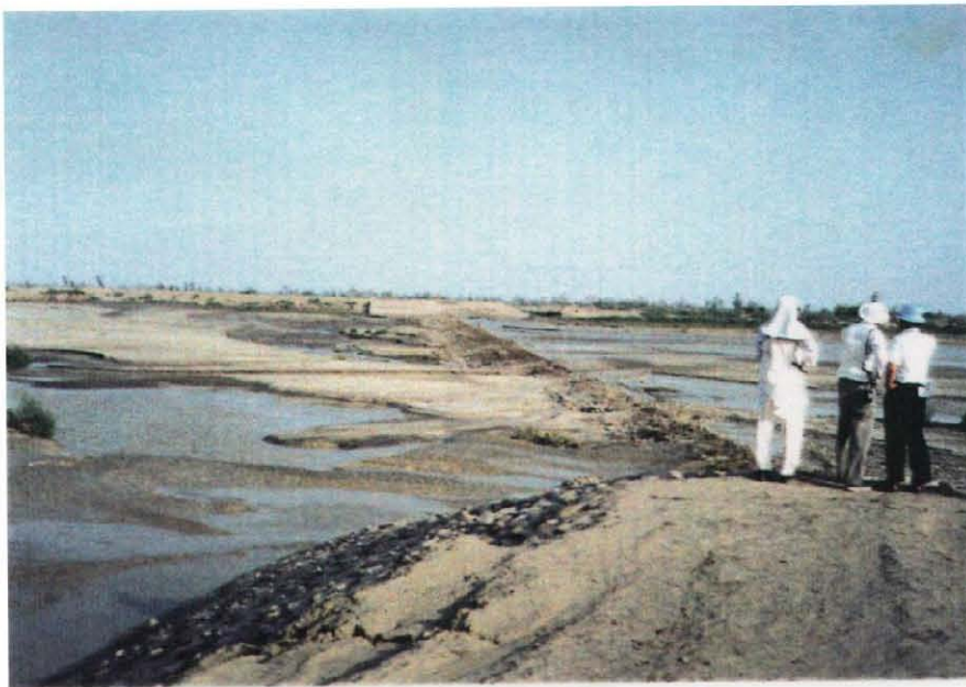
Intake & diversion weir
