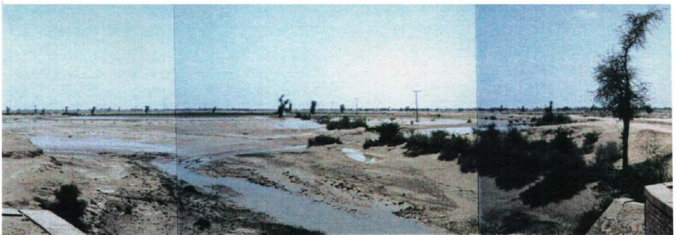
View of upstream from hill torrent diversing structure
