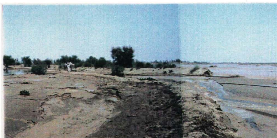
Diversion earthen bund
