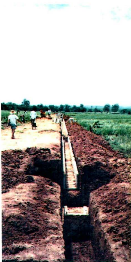
Rehabilitation of On-farm Canal 末端水路の改修
