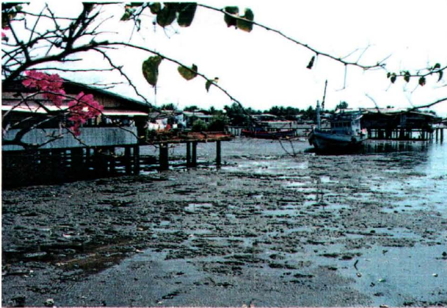
5. Grave situation of sedimentation at the outlet of Trat River
