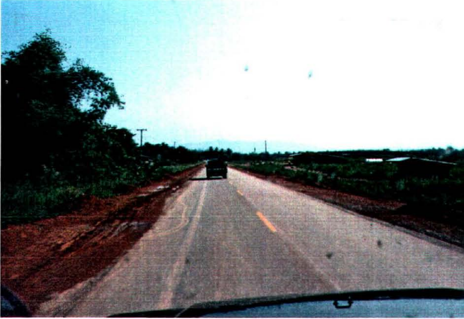
1. Access-Road to the Project-site
