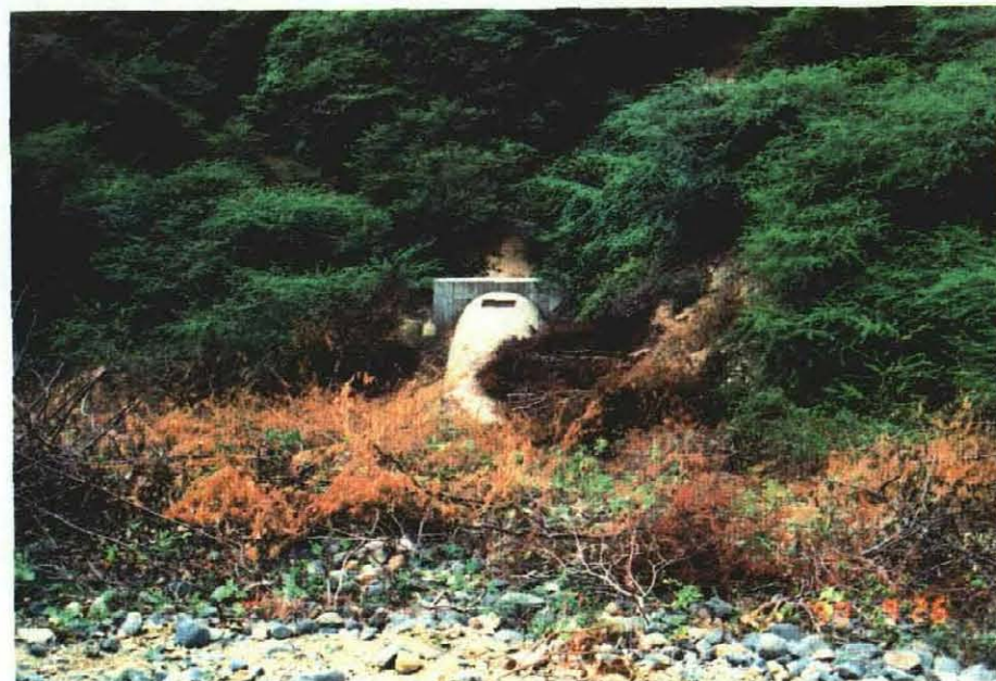
MAGUACA DAM, OUTLET AT THE DOWNSTREAM TOE
