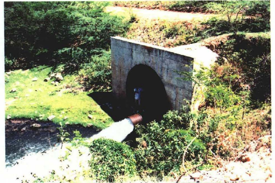
CHACUEY DAM, OUTLET AT THE DOWNSTREAM TOE AND EXISTING IRRIGATION CANAL
