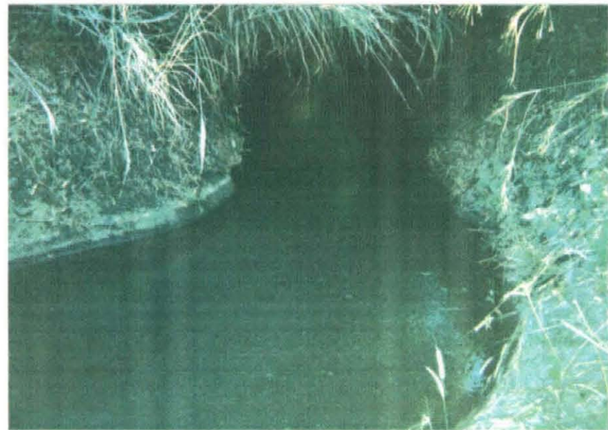
The Canal near the Existing Diversion Weir
