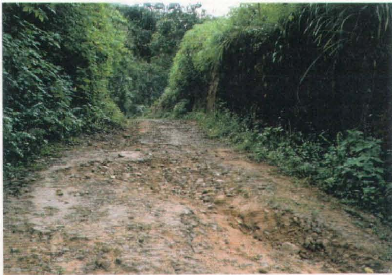
侵食対策の必要な農道 Farm road to be necessary for protection measures against sever erosion hazard
