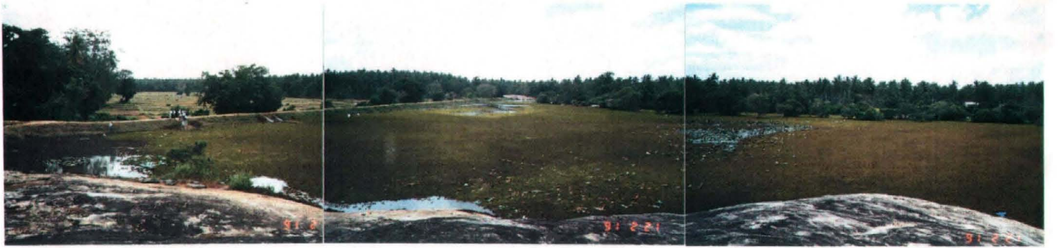
Ambewa Tank (1987 Rehabilitated)
