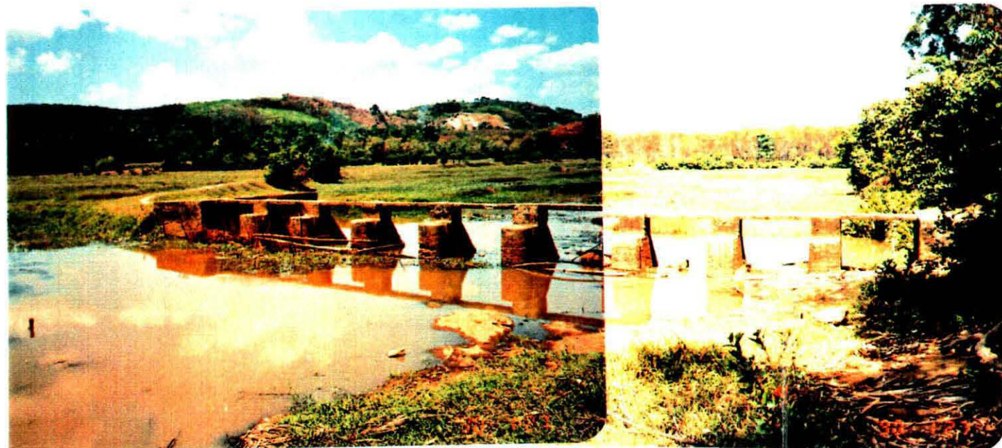
PITIYAGE WELA STRUCTURE
