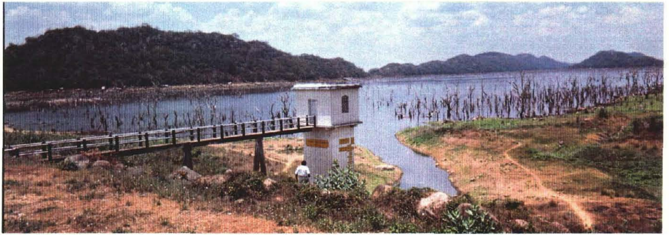
Wahalkada Tank (R.B. Sluice)
