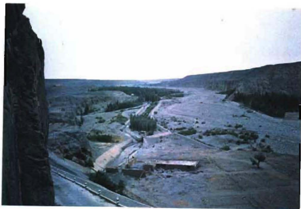
Downstream of Kuekuea dam The headrace canal has been lined in most part with wet masonry system.
