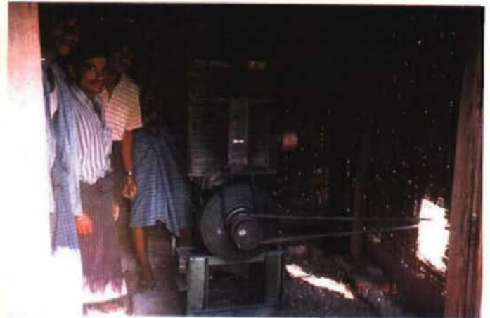
DIESEL ENGINE FOR WELL PUMP
