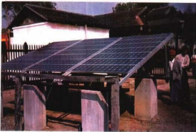
PHOTOVOLTAIC ARRAYS FOR WATER SUPPLY
