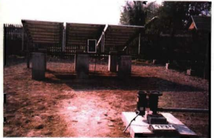
PHOTOVOLTAIC PUMP SYSTEM AT KAOGYI VILLAGE IN KYAUKSE TOWNSHIP, SAGAING DIVISION
