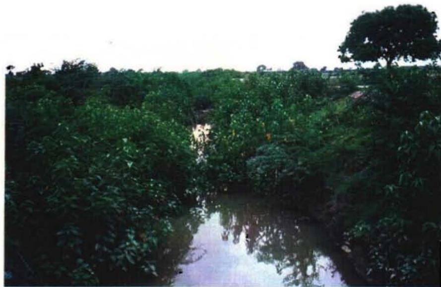
Heavy Weeds Population and Water Logging in Drainage Channels, Chambal Command Area, Rajasthan
