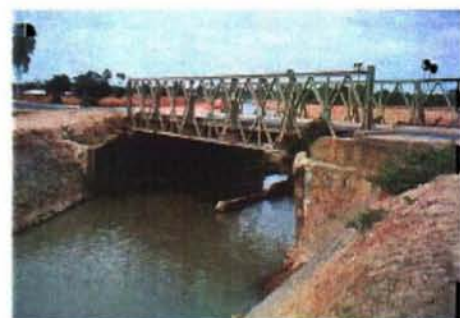
Kandal Stung Intake (to be rehabilitated)
