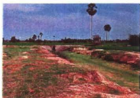
Existing Secondary Canal in the Existing Kandal Stung System (to be rehabilitated)
