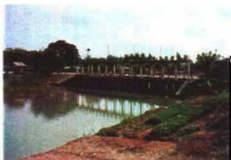
Tuk Thla Regulator (to be rehabilitated)
