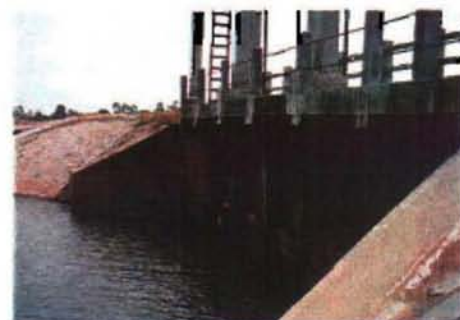
Kompong Tuol Regulator (to be rehabilitated)
