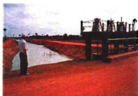
Stung Toch Regulator and Intake Channel (constructed in 1996/97)
