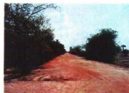
Connection dike cum road (to be rehabilitated)
