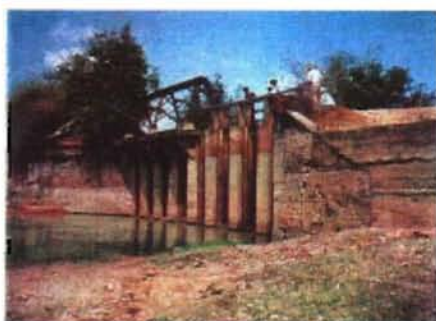
Regulator of Kpob Trobek main reservoir (to be rehabilitated)
