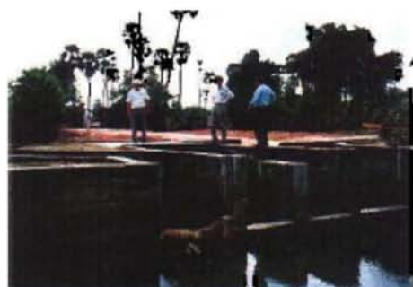
Bifurcation Structure in the existing Kandal Stung Canal System (to be rehabilitated)
