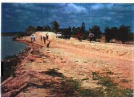
Dike of Tumnup Lok main reservoir (to be rehabilitated)
