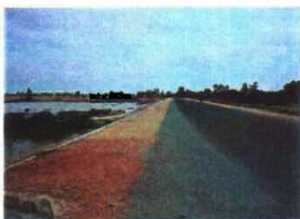
National Road No.3 Dike (Rehabilitated in 1996/97)
