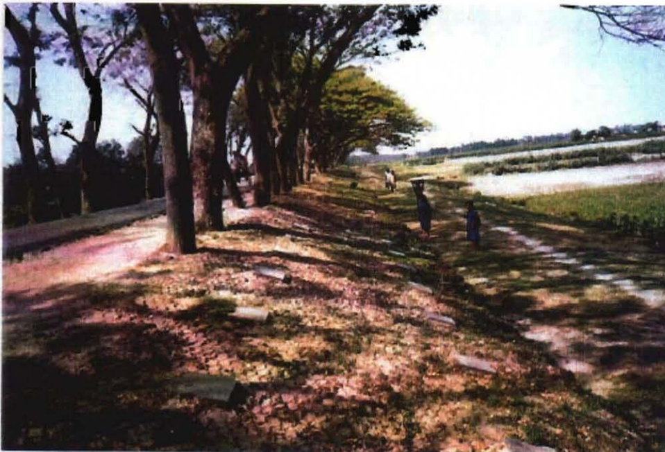
Slope protection of Gouripur - Homna Road
