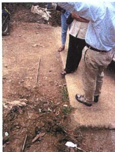
Municipality of Majayjay 配水管の布設状況
