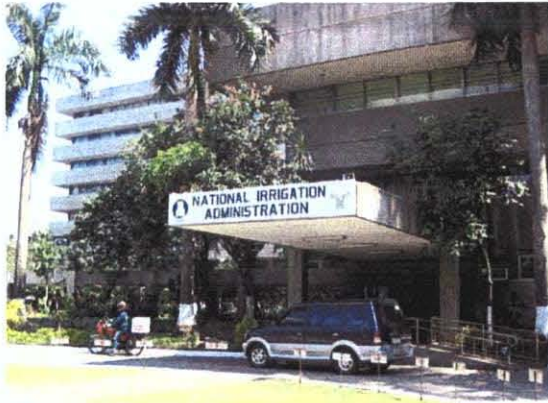
National Irrigation Administration 正面玄関
