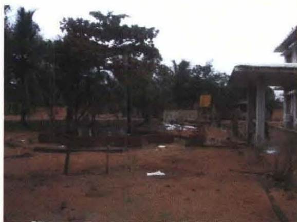
灌漑局事務所の被害状況 (バティカアラ県) Collapse of office building for irrigation department (Batticaloa)
