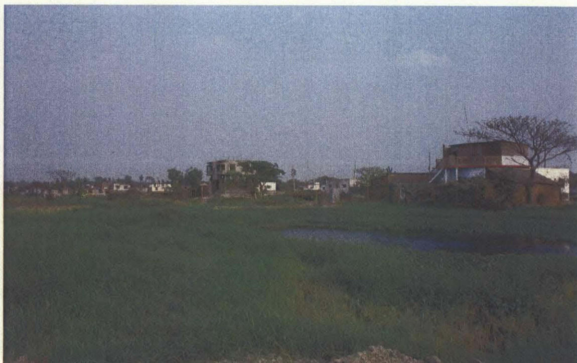
Drainage Canal Silted Up covered with Weeds
