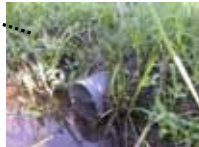
Outlet pipe at plot bund
